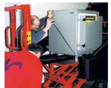
Professional installers moving a chamber kiln into a basement studio.
