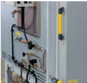
Gas supply system and thermocouple for automatic control system.
