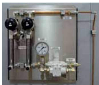
Gas supply system for HFL 160/17
