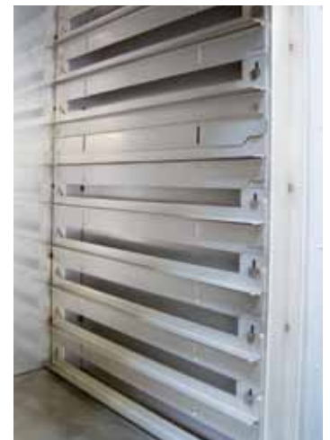
Adjustable outflow openings as additional equipment
